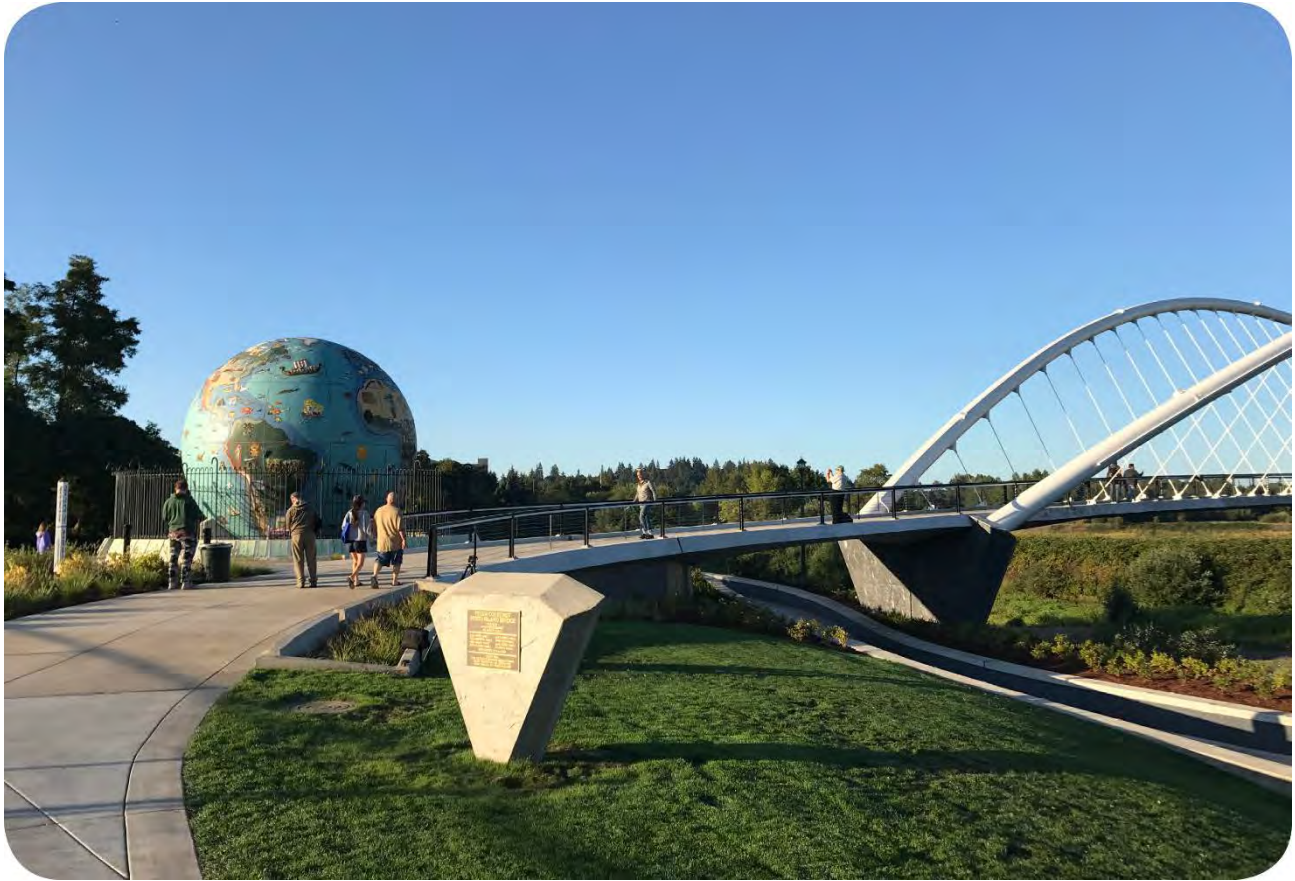
The Peter Courtney Minto Island Bicycle and Pedestrian Bridge opened in 2017.
